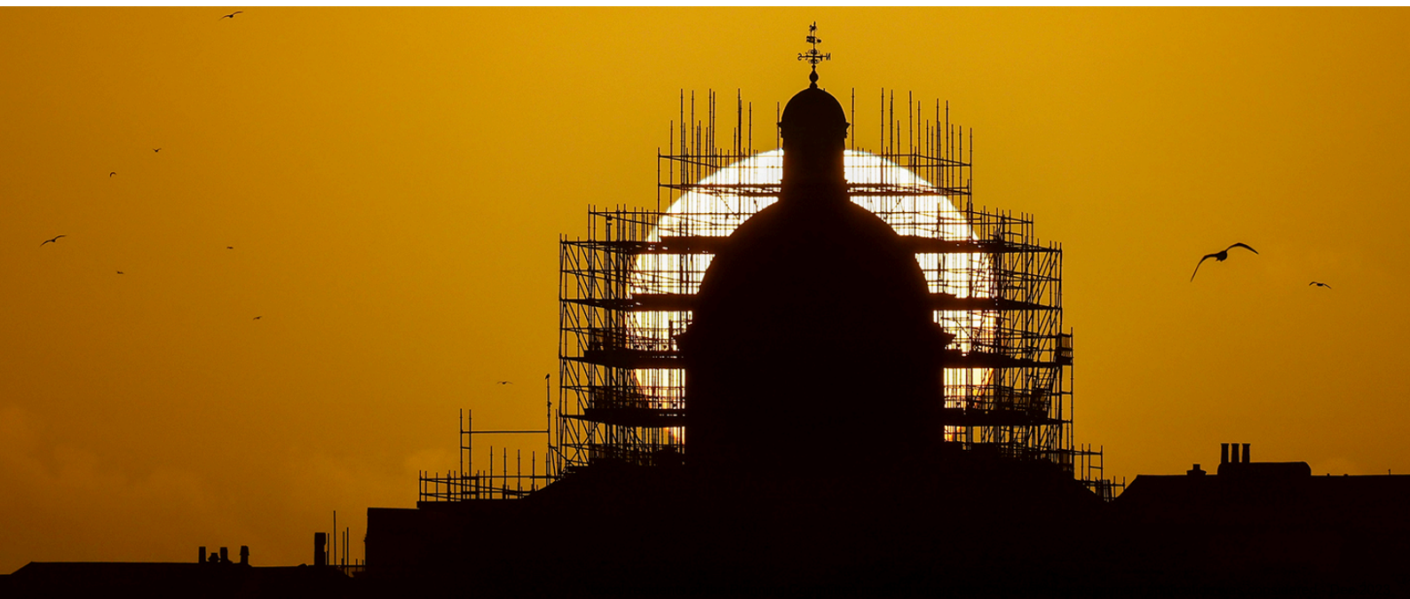
The sun sets behind the iconic dome of Market House during restoration works. Image: Greg Martin / Cornwall Live
