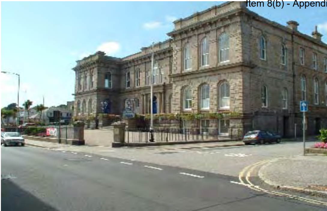
St John's Hall, is a monumental municipal building marking the edge of the commercial town centre, and the start of residential properties in Alverton Street
