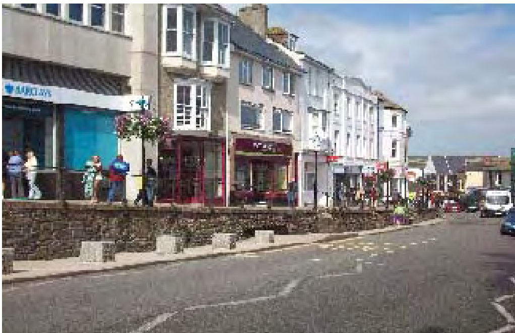
Generally buildings on the north side of Market Jew Street have survived better than those on the south side. The Terrace is particularly distinctive with its high quality granite paving, railings and steps.
