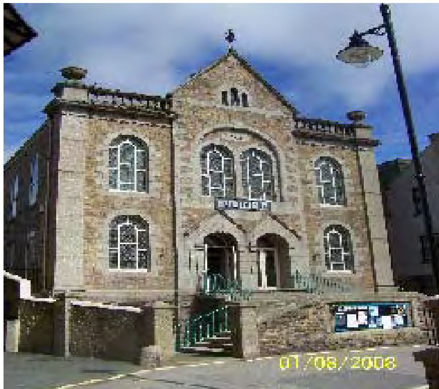
The Acorn Theatre stands as a successful non residential conversion redundant chapel within the town centre
