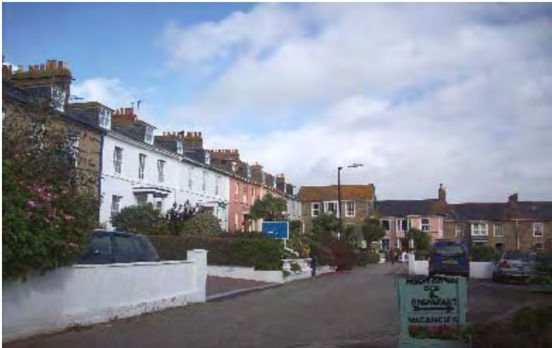
Regent Terrace, large Georgian properties used mainly as guest houses occupy an enviable position just off the Promenade
