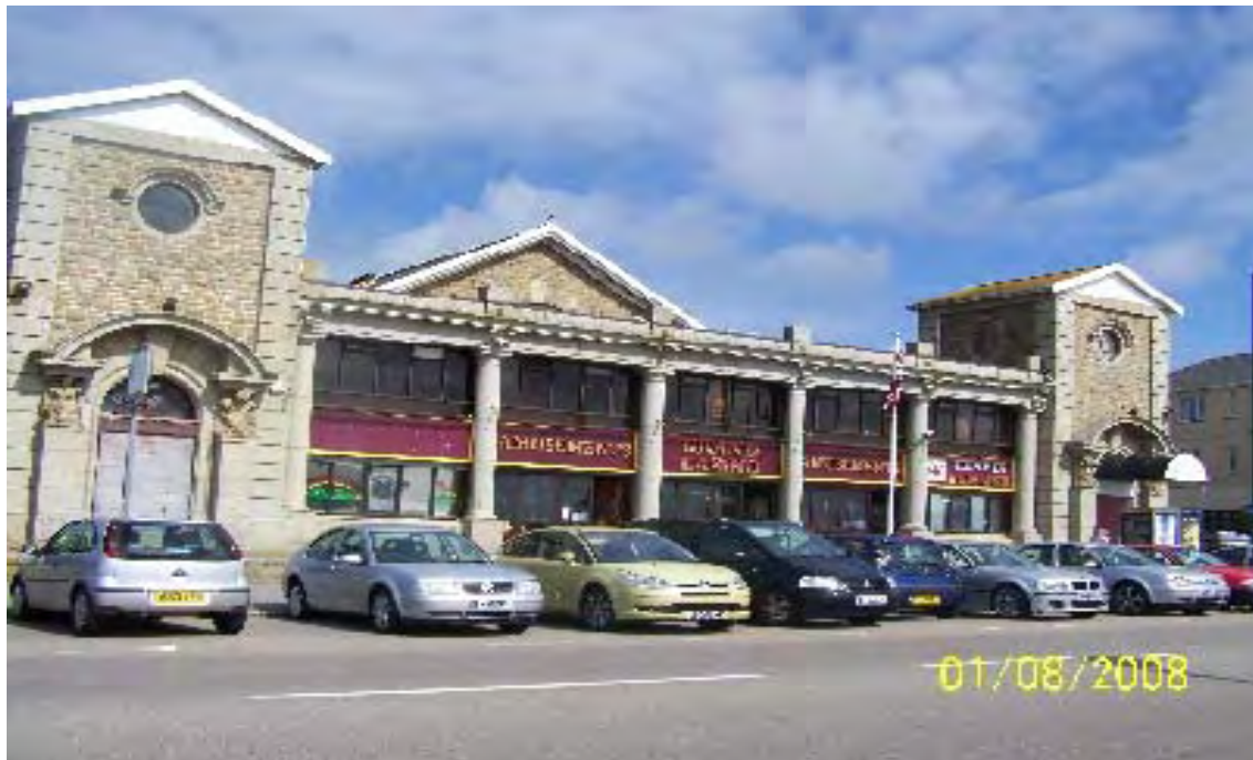
Parking dominates the front of the amusement arcade building, its lost its towers but still remains a local landmark, facing out to sea
