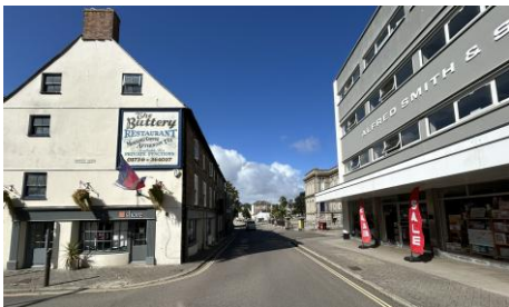
Figs. 31-34 From top to Bottom – Burinton House, Burinton House, site and Burinton House viewed from West, site and Burinton House viewed from East
