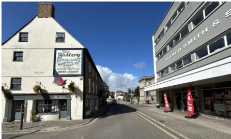
Figs. 40-43 From top to Bottom – First & Last Inn, First & Last Inn, site First & Last Inn viewed from West, site First & Last Inn viewed from East
