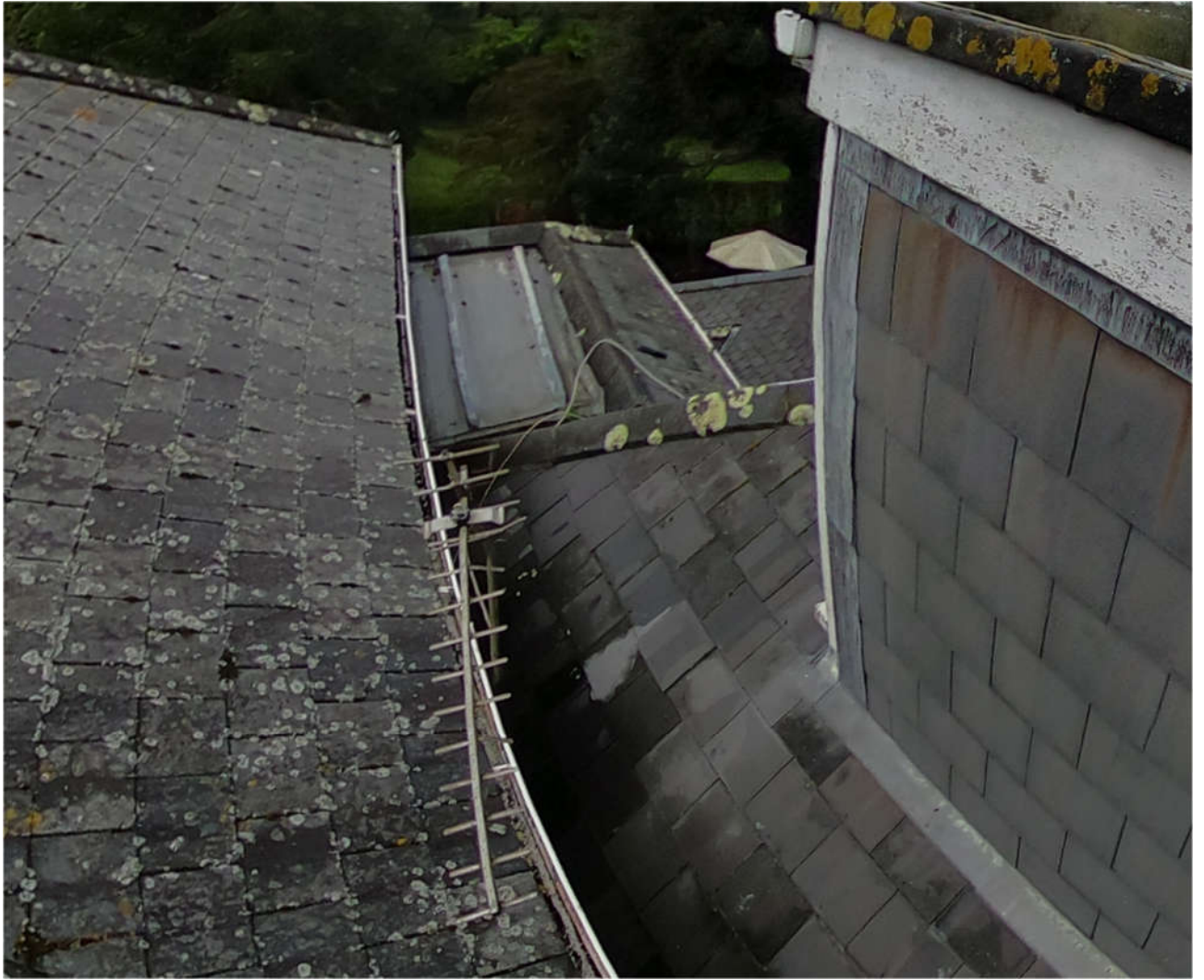
First Floor parapet roof
