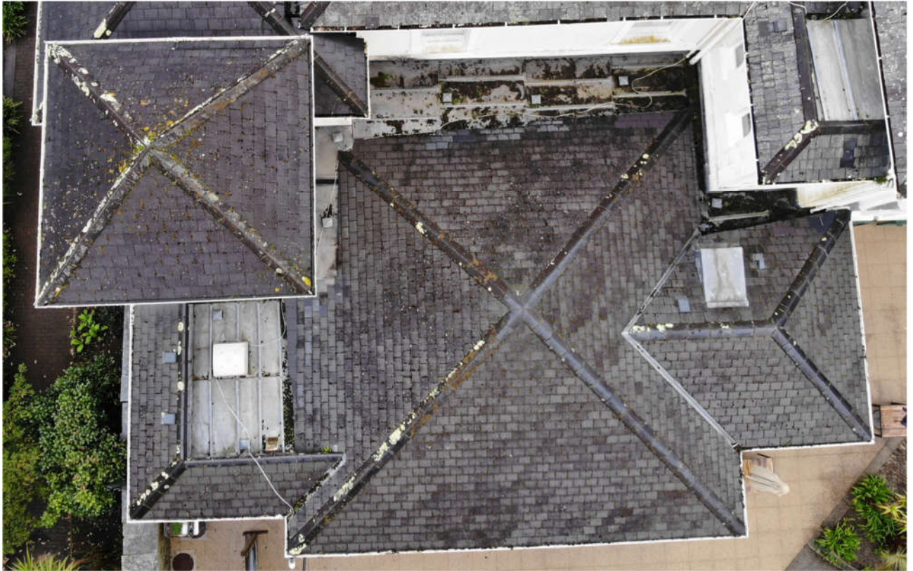
Ground Floor Roof
