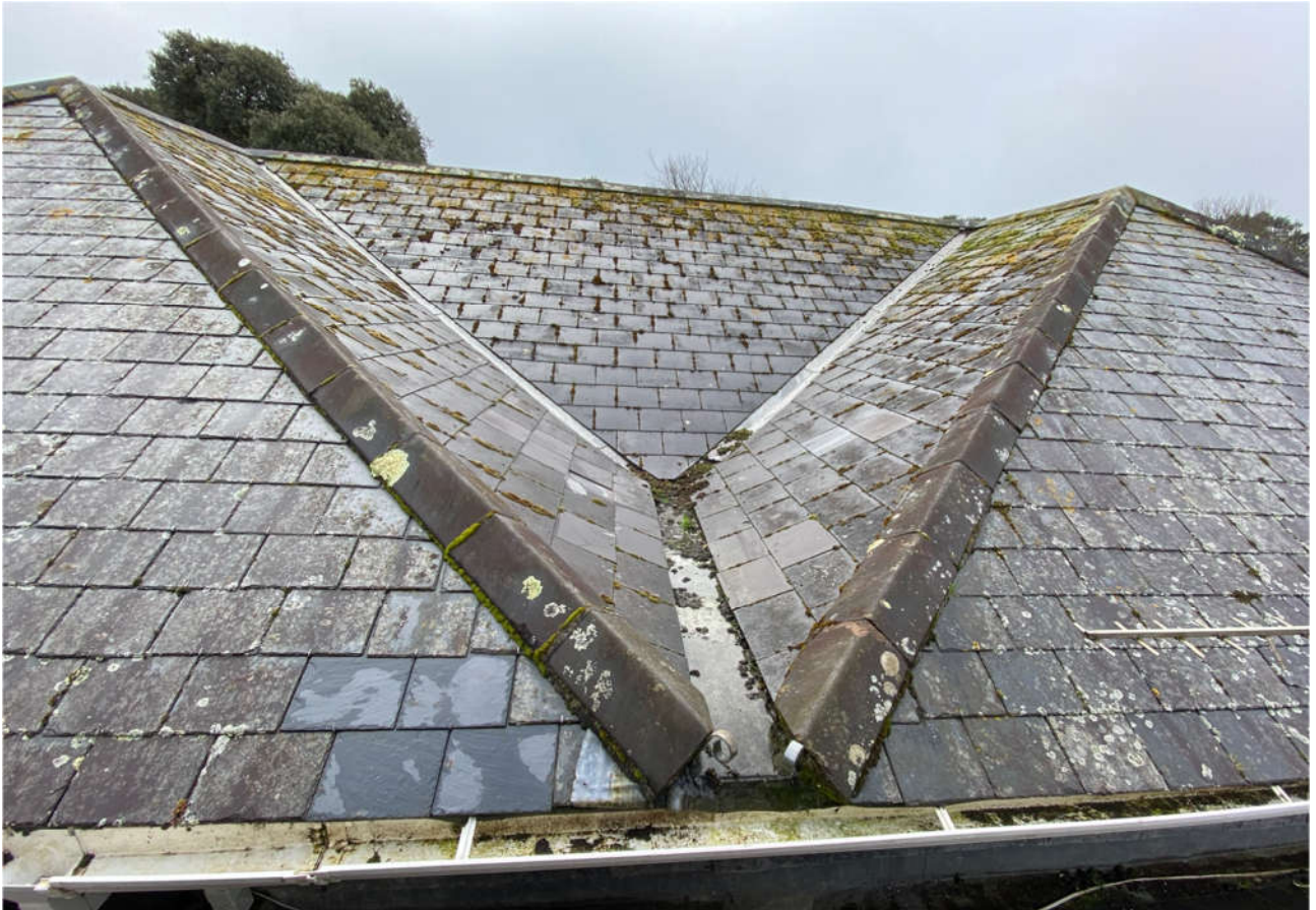
Main Roof and Valley
