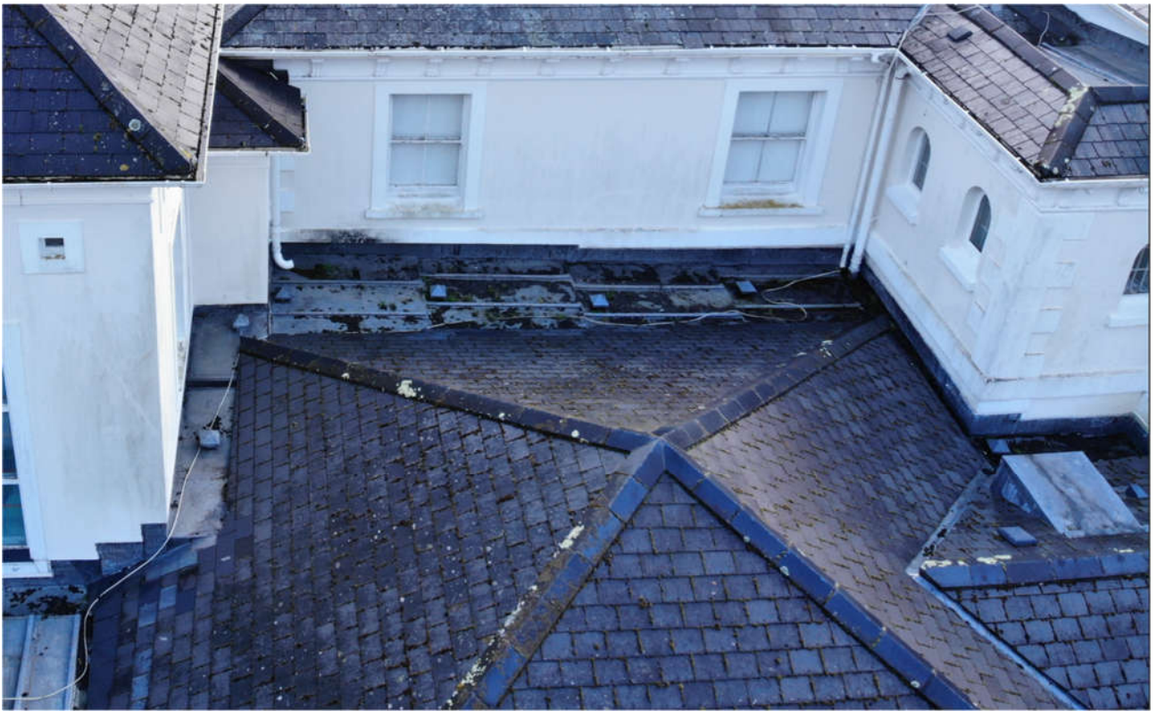
Ground Floor Roof
