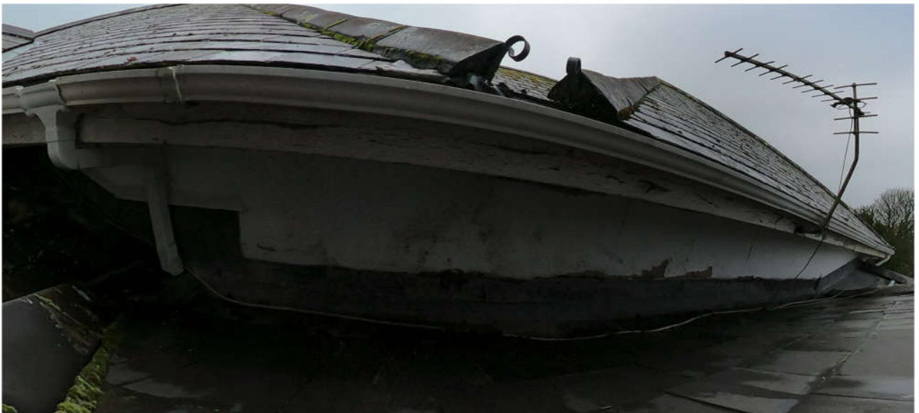
Box gutter below main roof valley
