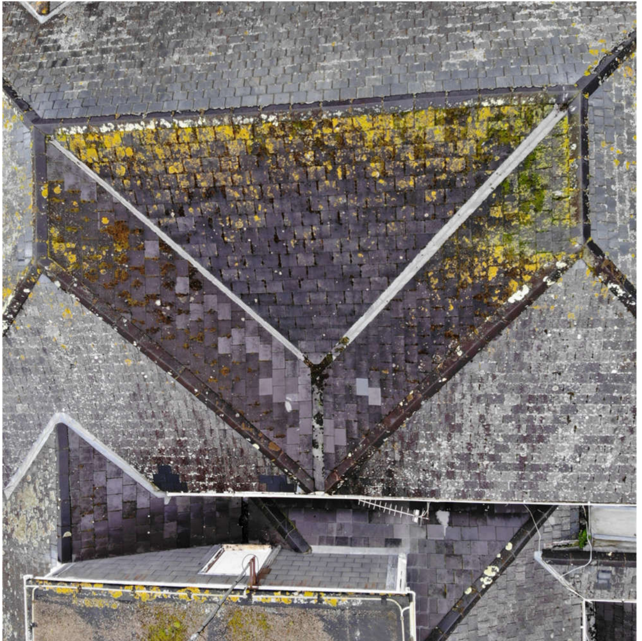
Main Roof and valley
