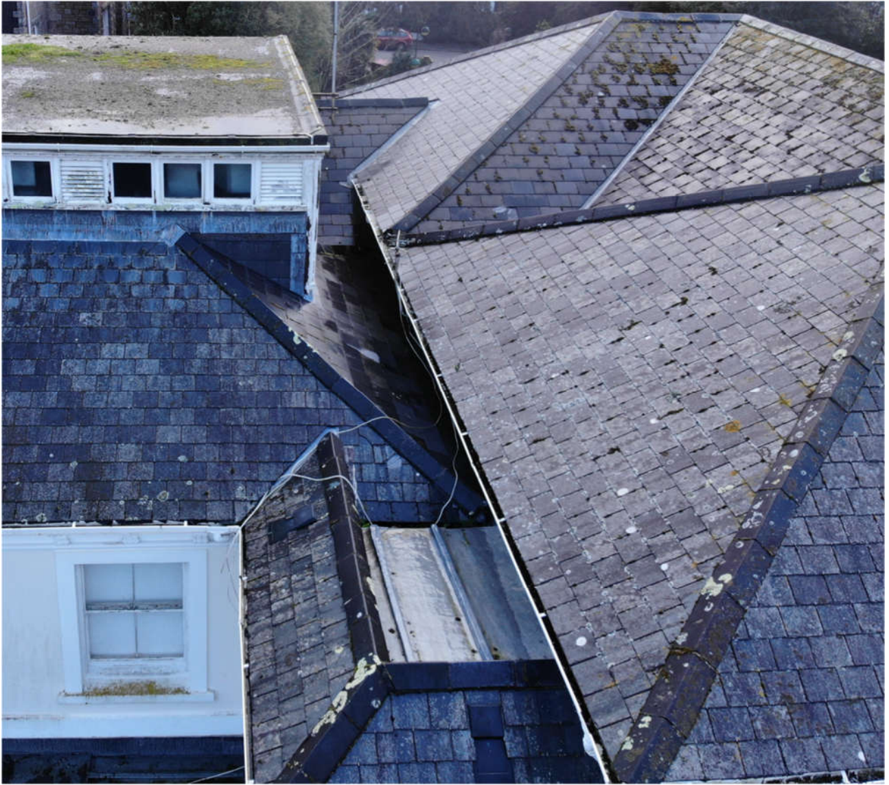
Main Roof valley, Box gutter and First Floor parapet Roof.
