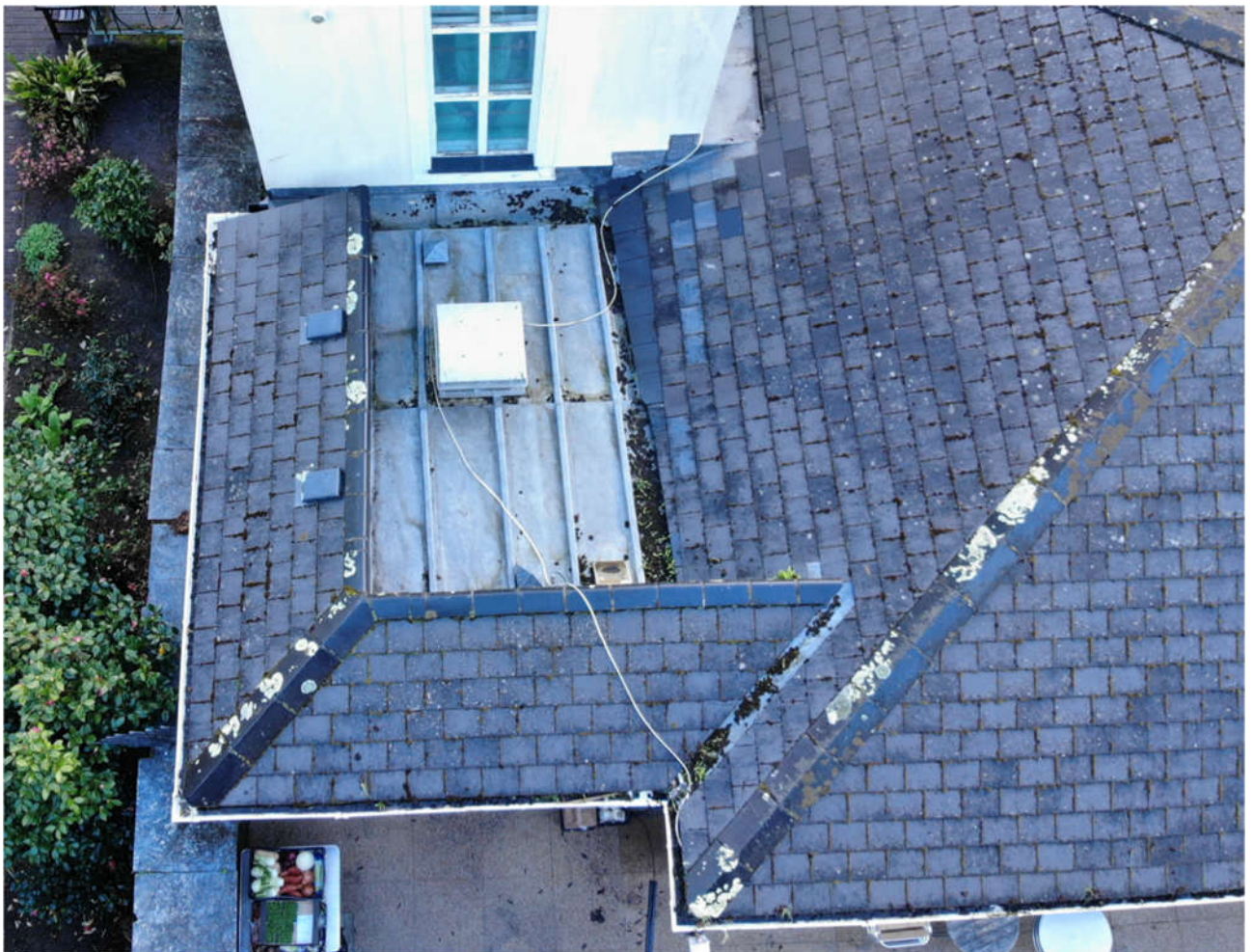
Roof above ground floor Commercial Kitchen
