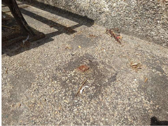
Old Bench Footing
