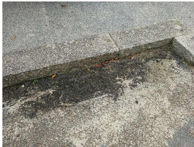
Existing drainage Gully (2024)
