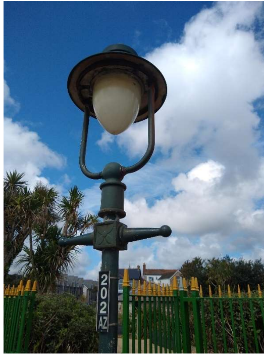
Typical Existing Column
