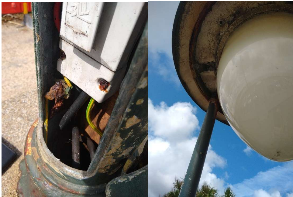
Existing Lighting Columns
