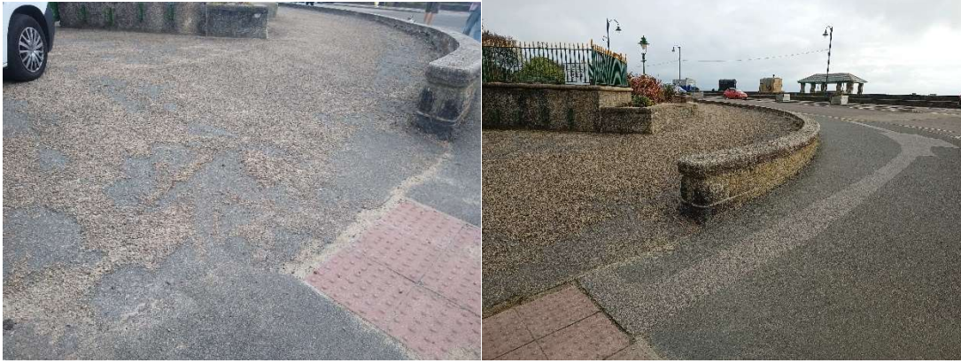
Start of Terrace at Alexandra Road (LH/2021 – RH/2024)
