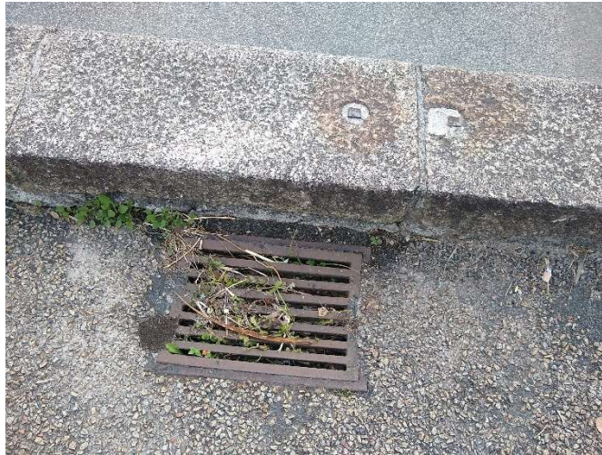
Existing drainage Gully (2021)
